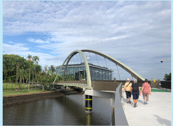
Breakfast Creek Green Bridge, completed in 2024.
