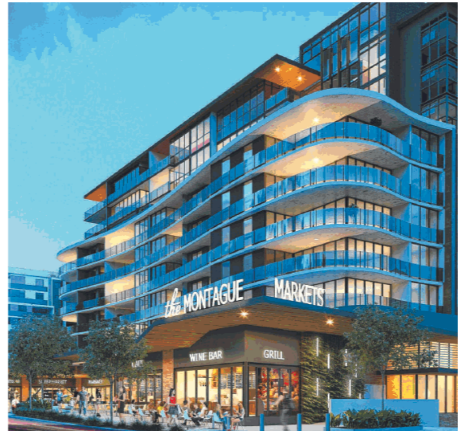
EXCELLENT FIT: An artist's impression of Pradella's $175 million mixed use West End precinct, Montague Markets and Residences.
